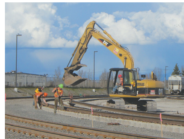
Rail work at Terminal 5
