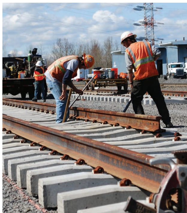
Construction crews at work on the port's rail project.
