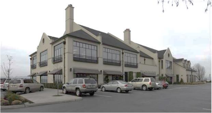
CE John Building
