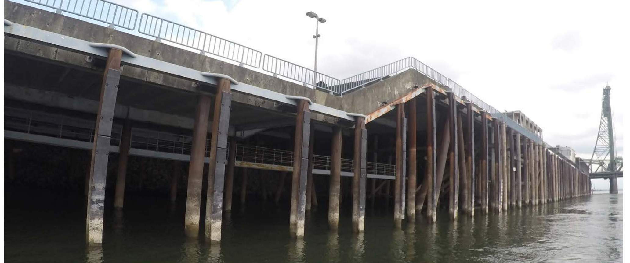
Figure 1.44 Concrete/Steel Pier Structure (west end, looking northeast)
