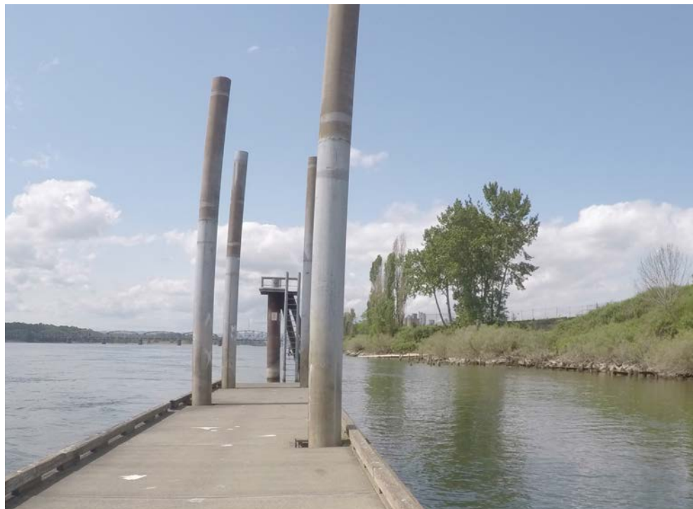
Figure 1.58 Low Dock (looking west)
