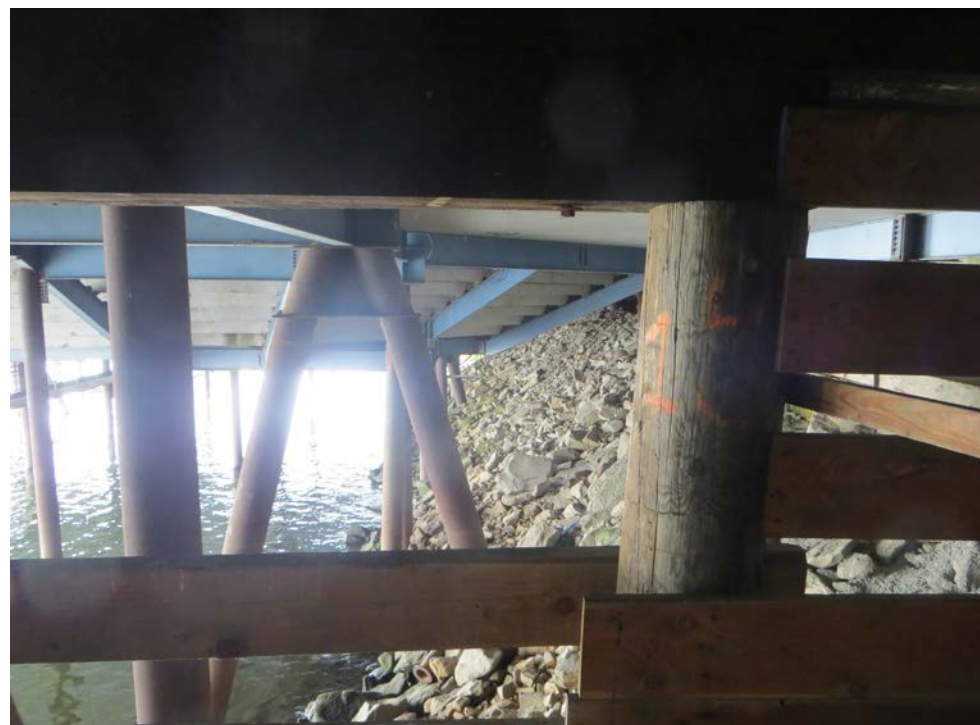
Figure 1.56 Pier Structure, Transition from Steel to Timber Pilings (looking west)
