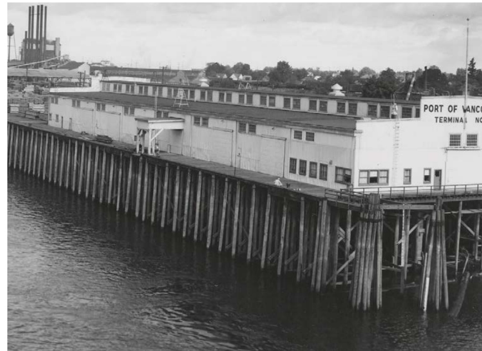
Figure 1.4 Terminal 1 Building, circa 1955 (south & east facades)
