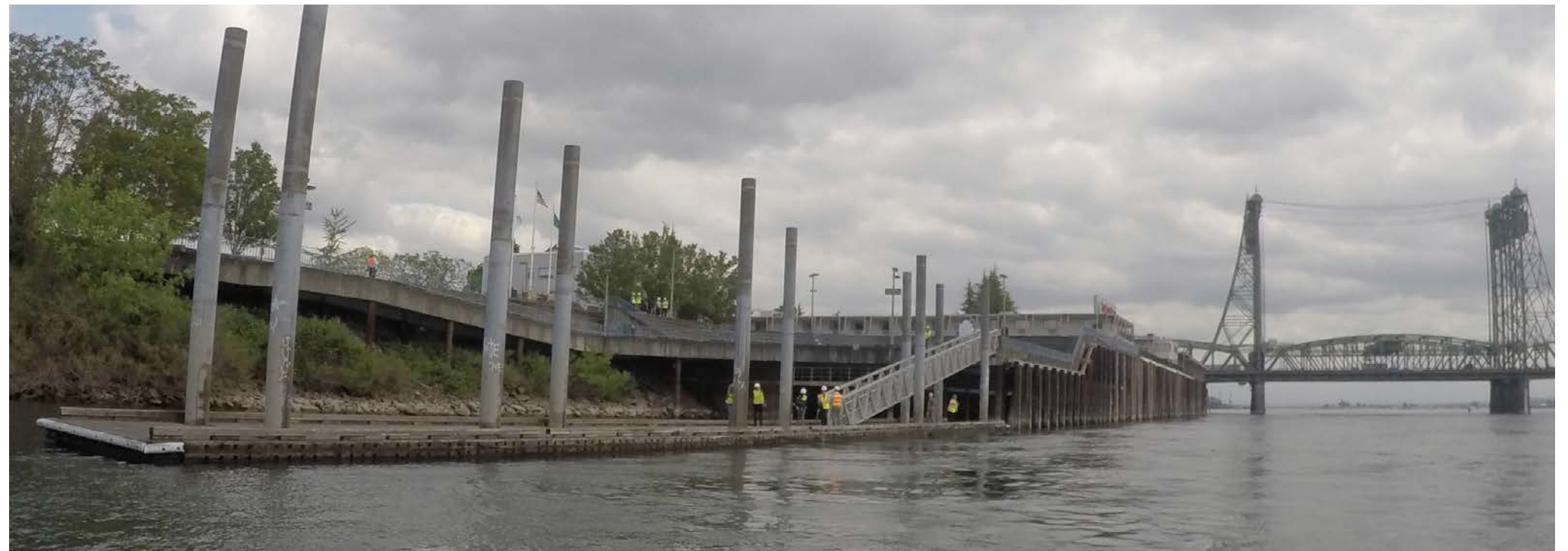
Figure 1.59 Low Dock & Terminal 1 Wharf (looking east)
