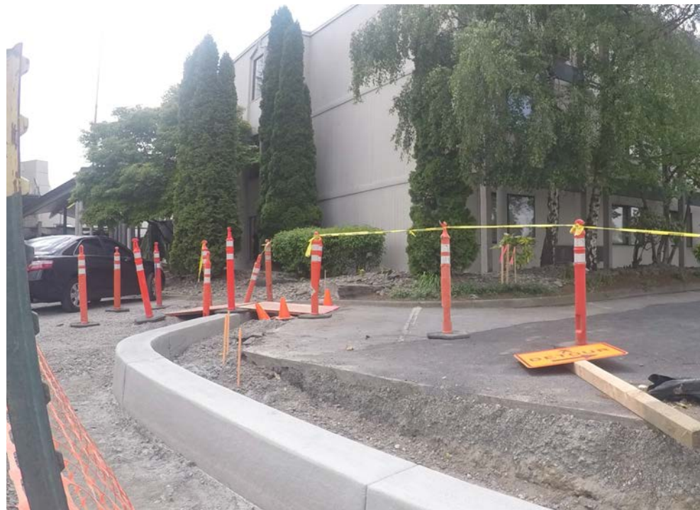
Figure 1.45 Columbia Way Construction, near Red Lion Hotel
