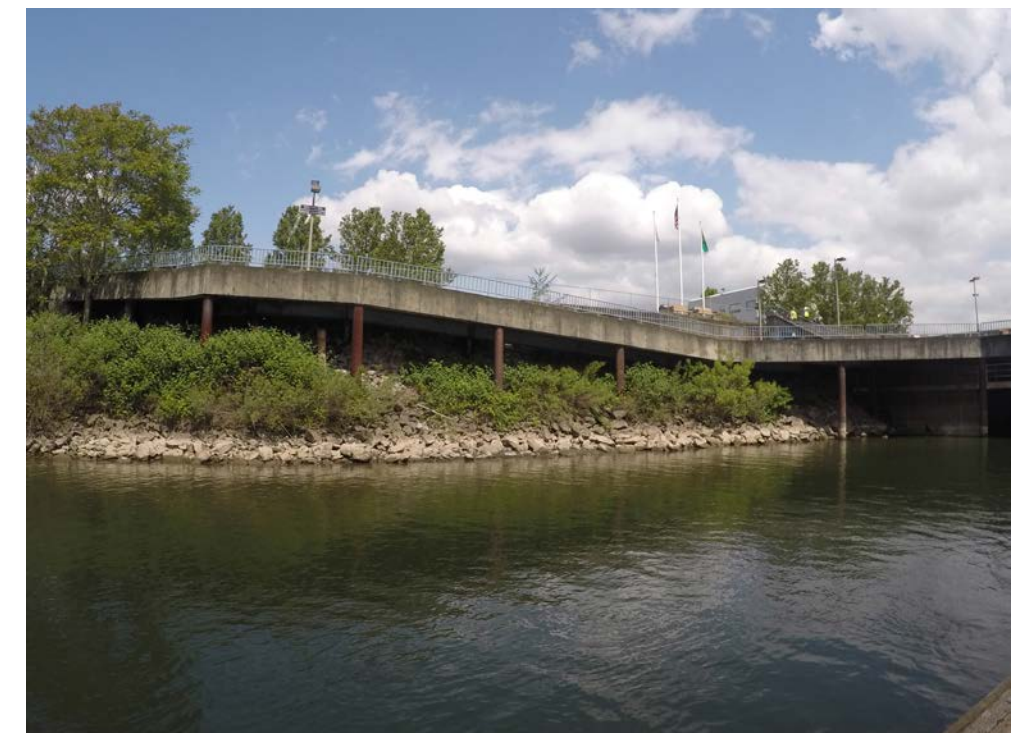
Figure 1.57 Shoreline Edge & Access Ramp (looking north from low dock)
