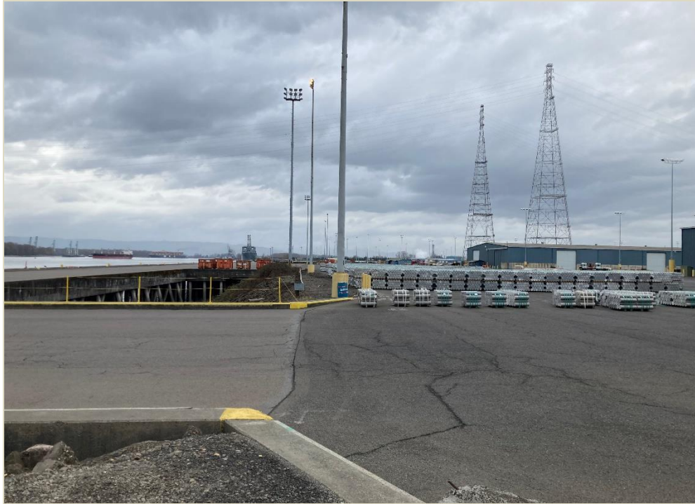
Photo 6. At the time of inspection, aluminum ingots were being stored where there will be deep soil mixing north of Berth 8, which is on the left. The gap between the upland and overwater portions of Berth 8 will be filled. The view is towards the northwest.
