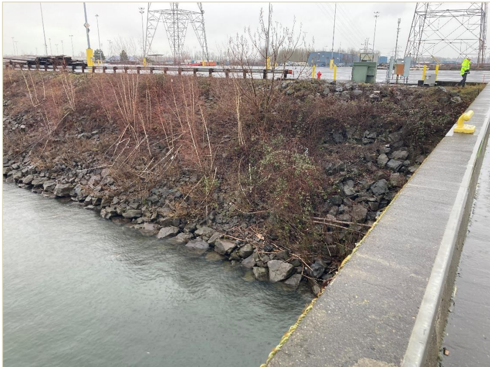
Photo 5. Rip-rap armors the portion of filled shoreline where the Port will construct the downstream extension to Berth 9. The footings of the Ross-Rivergate No. 1 and Ross-St. Johns No. 1 transmission line towers are visible in the background. The view is towards the northwest from the current western edge of Berth 9.
