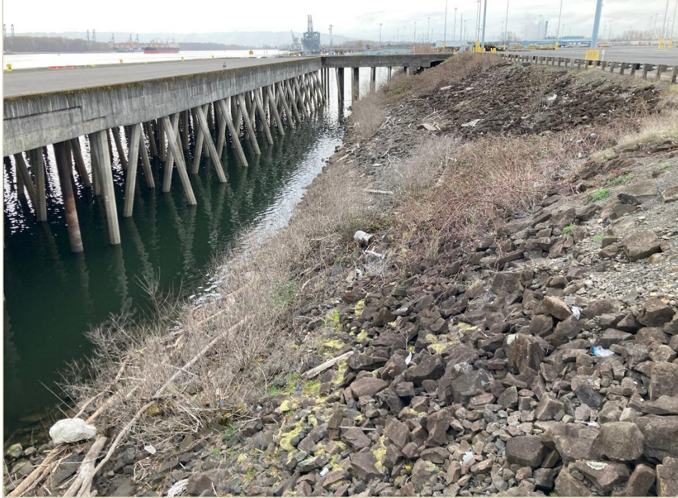
Photo 2. The gaps between the upland and overwater portions of Berths 8 and 9 will be filled as part of the project. The view is towards the west. Photo courtesy of the Port of Vancouver.
