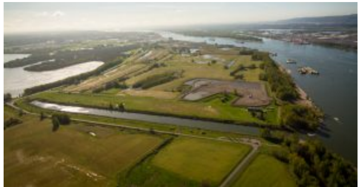
The flushing channel connects Vancouver Lake (left) and the Columbia River (right) to funnel fresh water into the lake to improve circulation.
